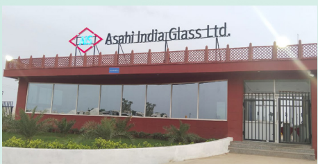
Float Plant- Soniyana Rajasthan
