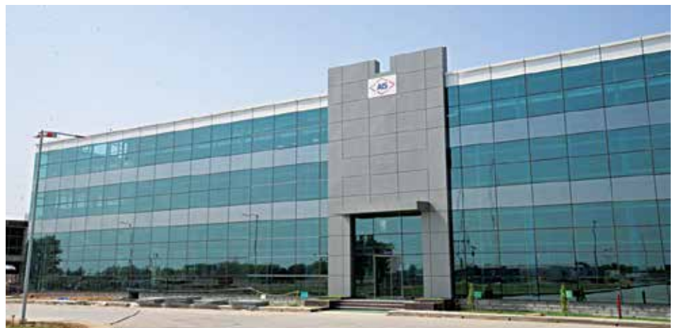
AIS Auto plant in Patan, Gujarat, has received the esteemed IGBC Green Factory Buildings Rating System - Gold certification
