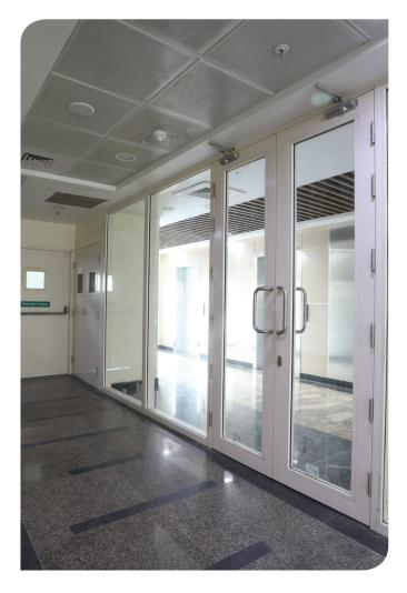
as a transparent barrier, providing visibility and natural light transmission while ensuring fire protection. Firerated glass withstands extreme heat, restricts heat
