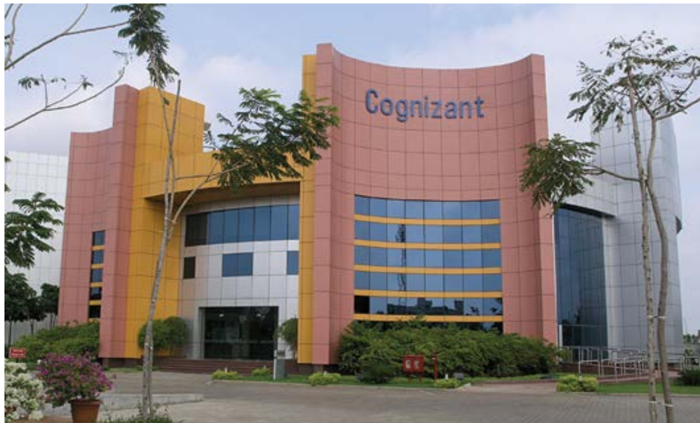
CTS Headquarters, Thoraipakkam, Chennai by CRN Architects
