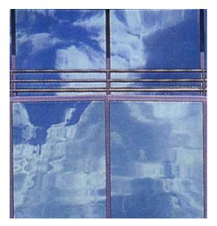
Figure 2: Architectural example of Optical Roll Distortion in Heat-Treated IG
