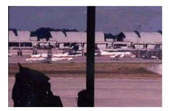
Figure 3: Architectural example of Optical Roll Distortion in Laminated Window
