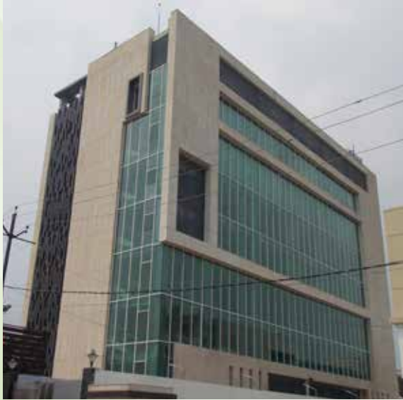
Bajaj Bhawan, Lucknow 6 mm Clear Essence – 12 mm Air Gap – 6 mm Green Tinted with Ceramic Frit
