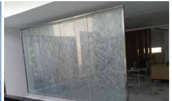
Residence in Bengaluru AIS Fabric-Laminated Glass
