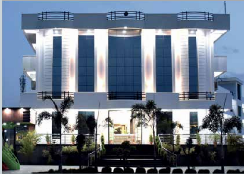
Project Name: Shiv Jyoti Convent School City: Kota, Rajasthan Product used – Façade: Opal Pearl Grey, 5 mm thickness
