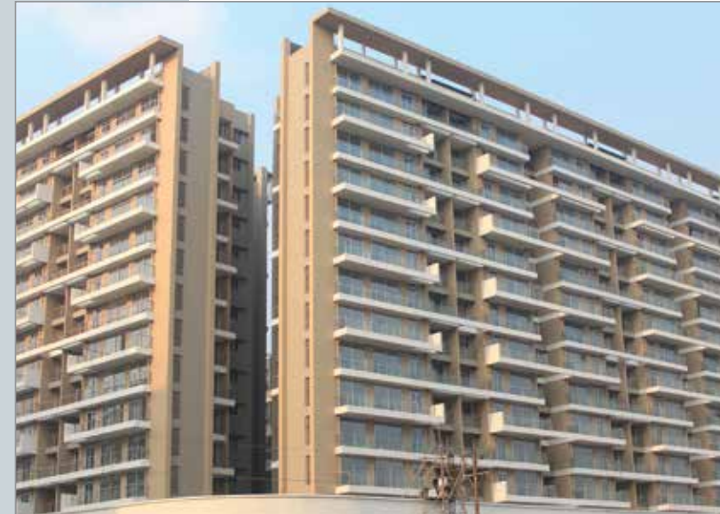
Project Name: Mayuresh Delta City: Ulwe, Navi Mumbai, Maharashtra Product used – Façade: Sunshield Clear, 4 mm thickness
